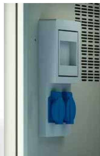
Socket outlet 230V / 16A with cover, FI/LS switch per compartment
